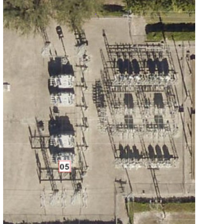
05-Lehigh Existing A-Bus
