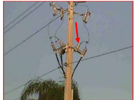
Infrared inspections detect hot spots. The equipment can be replaced before it causes any interruptions.
